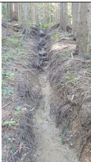
Obrázek 3: Surface ditches implemented in the upper part of landslide Betel (Jesenice, Slovenia) (Archive GeoZS).
