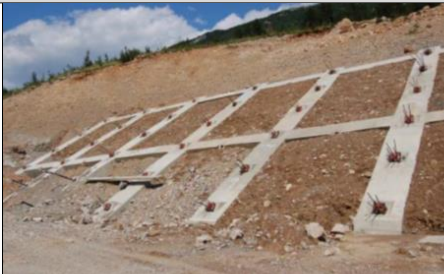
Obrázek 10: Anchored reinforced concrete frame on highway Razdrto-Vipava (landslide Rebernice, Slovenia) (photo B. Pulko).
